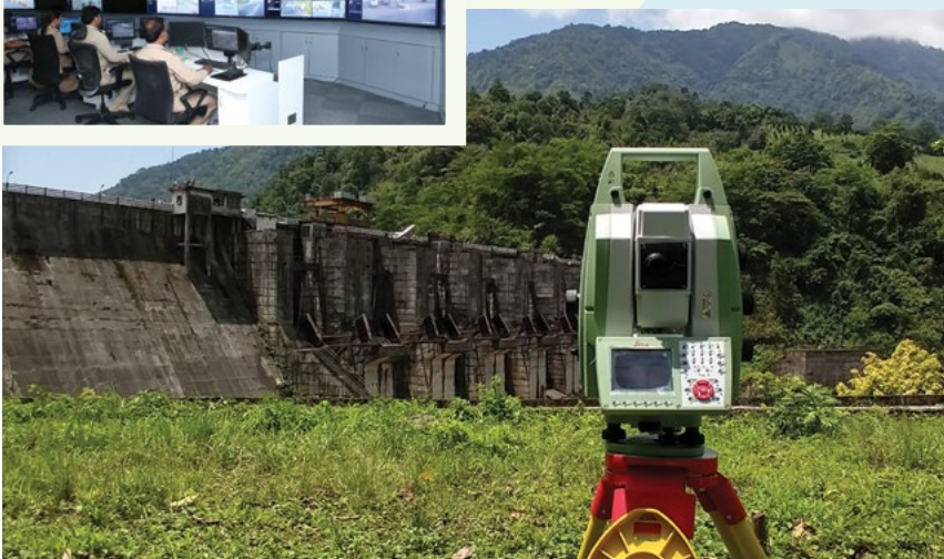
Below: Structural Monitoring of Neepeo Ranganadi Dam
