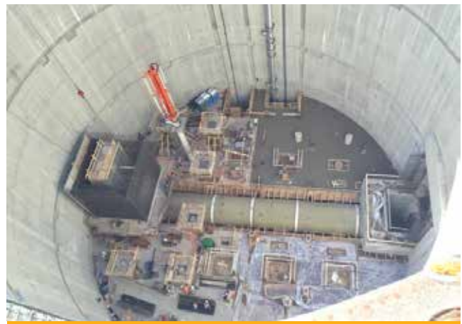
»» Installation of large components (the pipe is 13 feet in diameter) relied on precise measurements and accurate modeling. Scans of shaft walls captured beam pockets and keyways for future floors.
