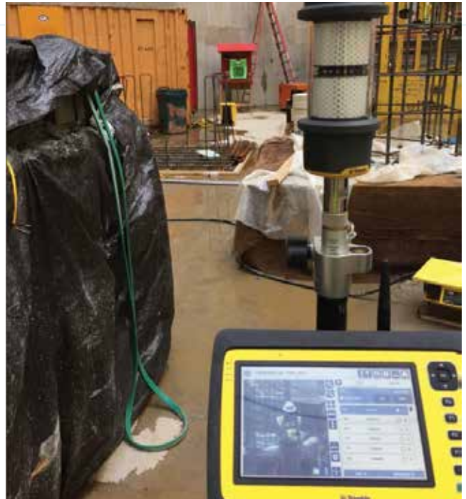
»»» A PC surveyor is shown on the Yuma display. The surveyor is seen from the total station mounted on a bracket on the shaft wall (above the red ladder.)
