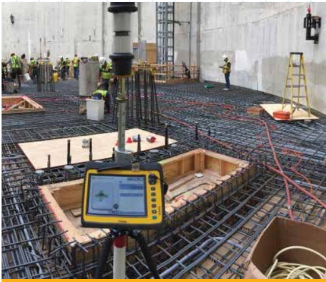
»» The view from the prism pole during layout. The display guides the user to the correct location. Brackets on the shaft walls hold prisms for control points. The total station is visible above the workers to the left of the prism pole.
